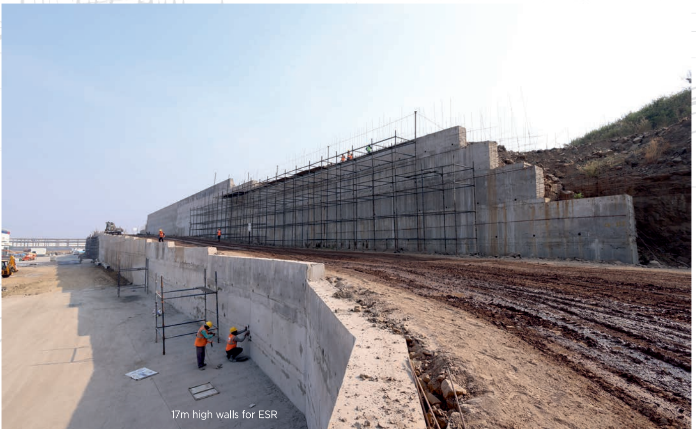
High-Rise Backfill Retaining Walls for TATA Group
