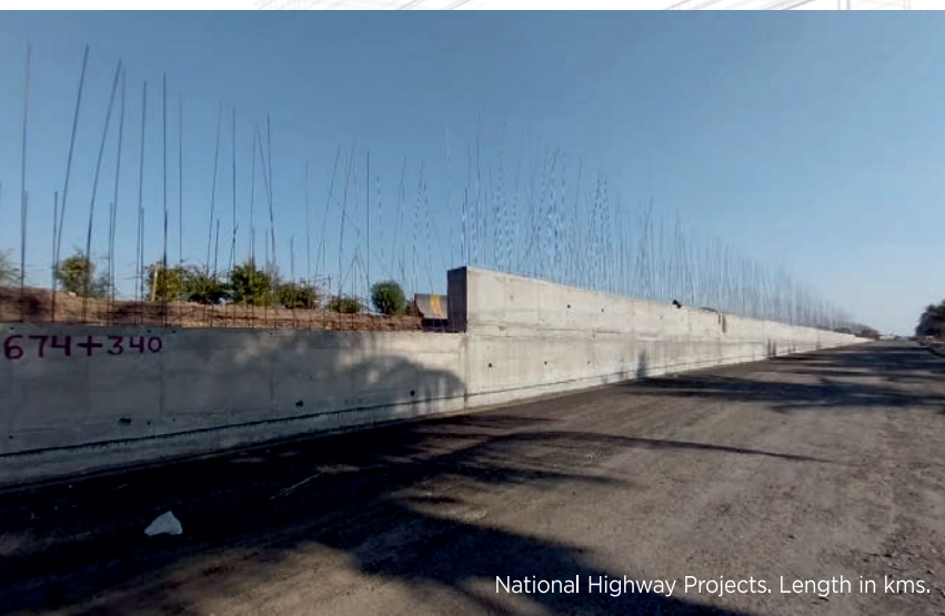
9m high walls for ROB of Central Railways.
